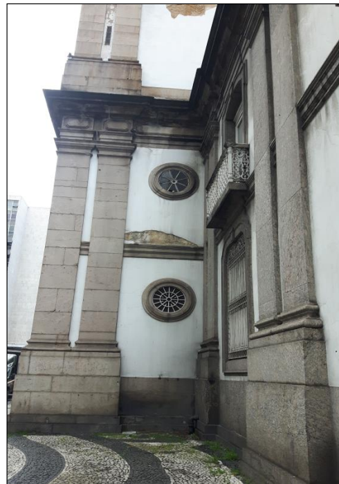
Figure 3. Columns of Facoidal gneiss (right) and Leptinito (left) of the Candelaria Church and Portuguese pavement. Photo: Nuria Castro (2019).
